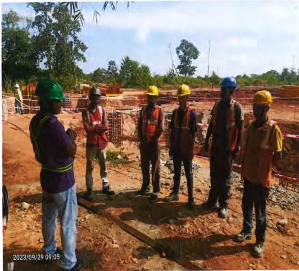
Photos of tool box talk on Gas cutting safety
