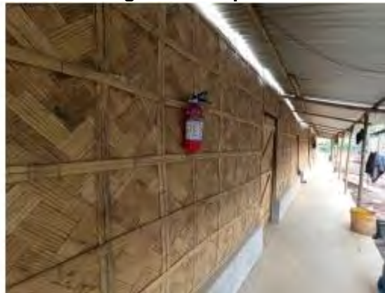
Fire extinguisher placed in labour camp CP-1
