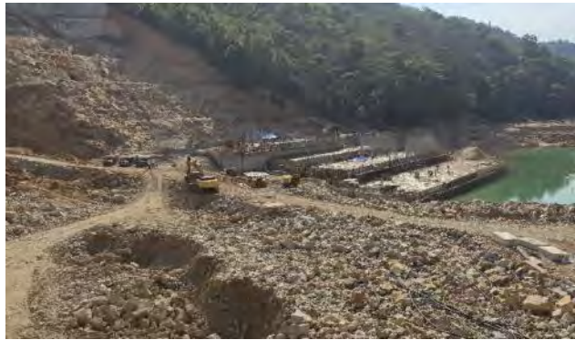
Left abutment and first layers of Blocks 6 to 10
