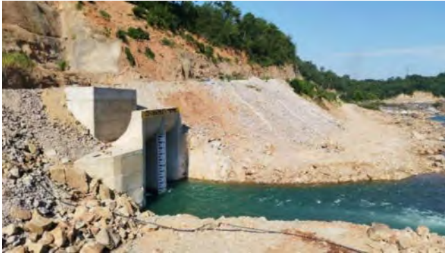
Intake to the diversion tunnel
