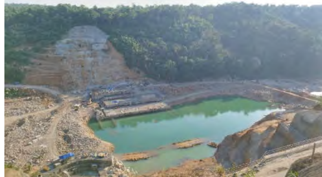
General view of dam, cofferdams and left abutment
