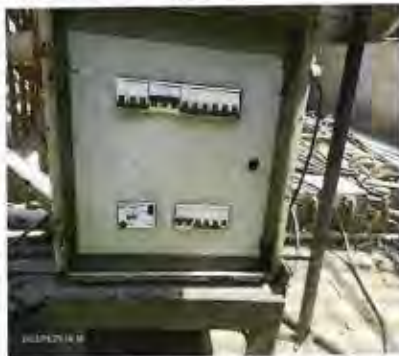
RCCB has been replaced.
