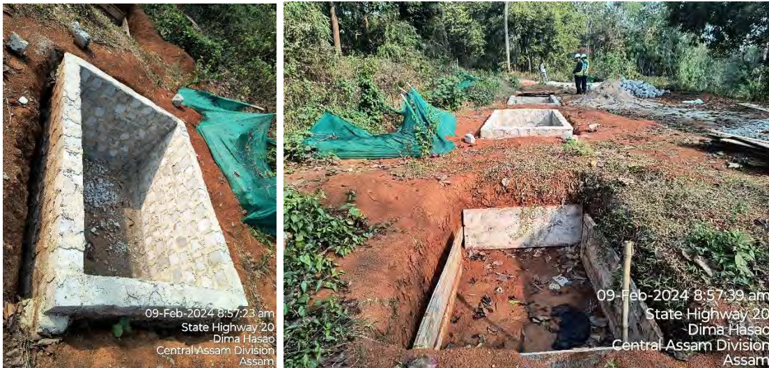
Compost pits constructed. Use of cement cubes after testing
