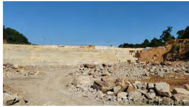
Downstream of the upstream concrete cofferdam
