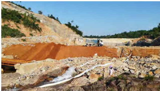
View of the downstream cofferdam with soils to improve impermeability
