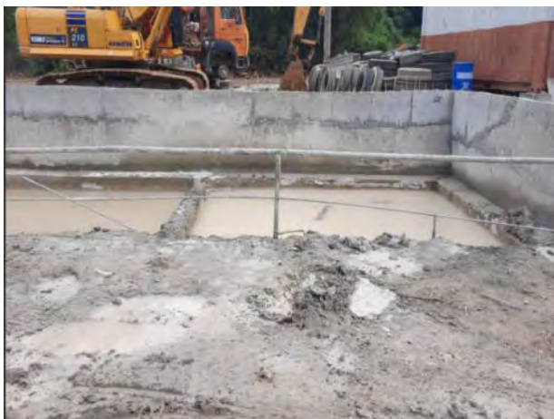
Batching Plant area - Sedimentation tank requires improvement
