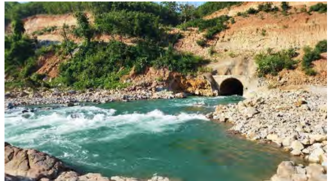
Final section of the diversion tunnel
