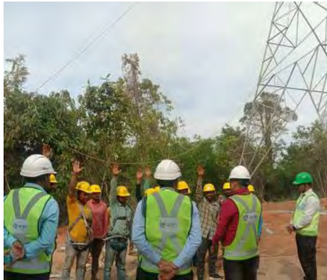
Pkg-4 - Tower Erection Site – Tool Box Talk. Dec 23
