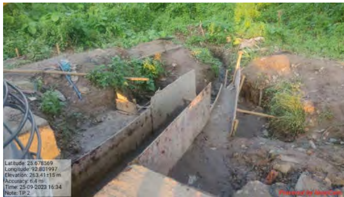
Vehicle wash and maintenance facility by package 2 contractor
